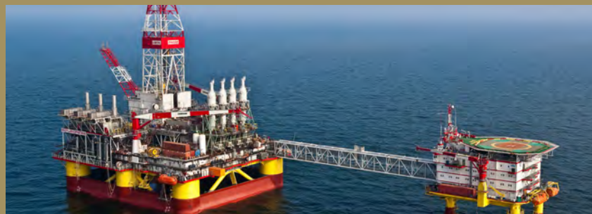
LSP-1 ice-resistant fixed platform on LUKOIL's Yuri Korchagin field in the Caspian Sea
