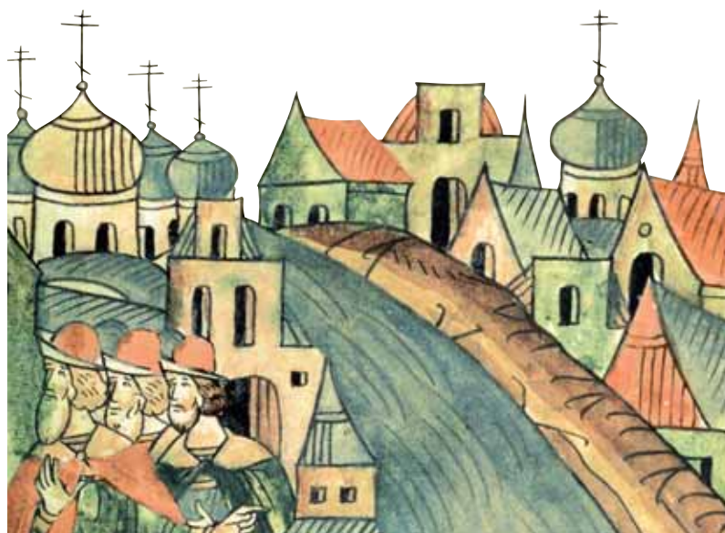
CONSTRUCTION OF A DITCH RUNNING FROM THE BORO- VITSKAYA TOWER, 1493
