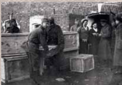
On October 12 th , 1941 upon the order of State Defense Committee at the Kashirskaya GRES was begun deinstallation of equipment and yet on October 14 th to Novosibirsk were sent first trains with boilers and turbines. During two months were sent around 500 wagons.
