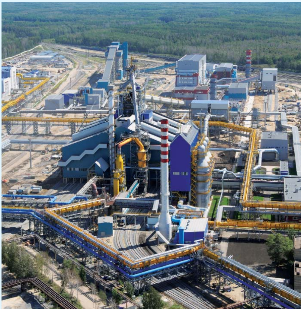
The Blast Furnace #7 is considered to be one of the most efficient facilities in the world
