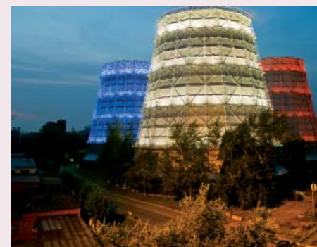
VIZ-Stal is a rolling mill that produces grain oriented (transformer) steel.
